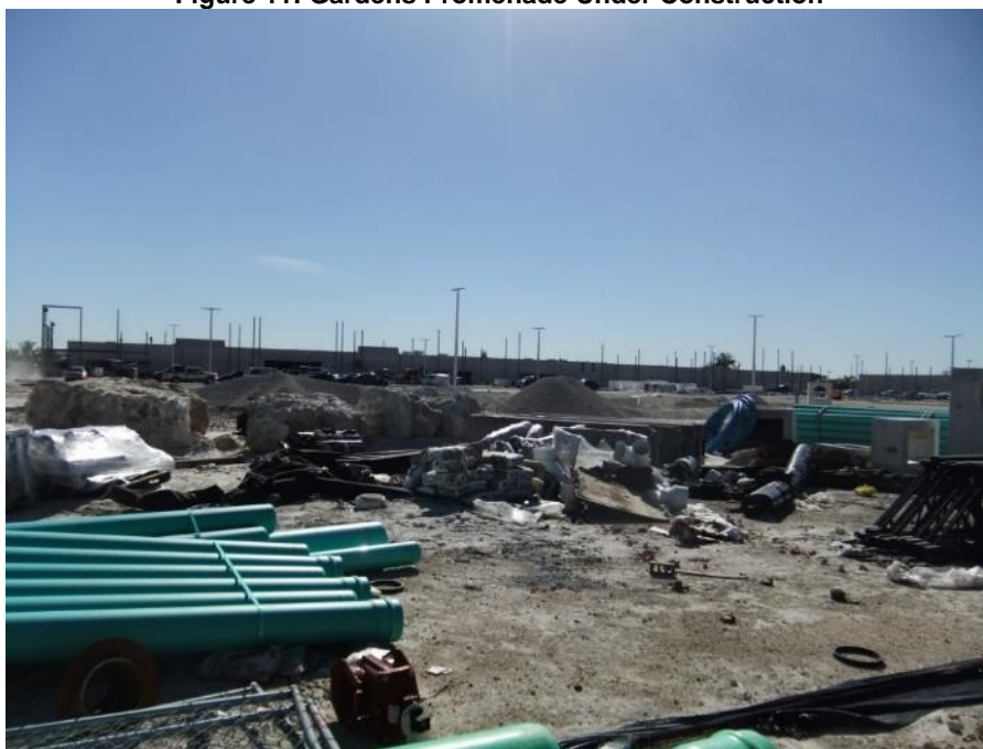
Figure 11: Gardens Promenade Under Construction
