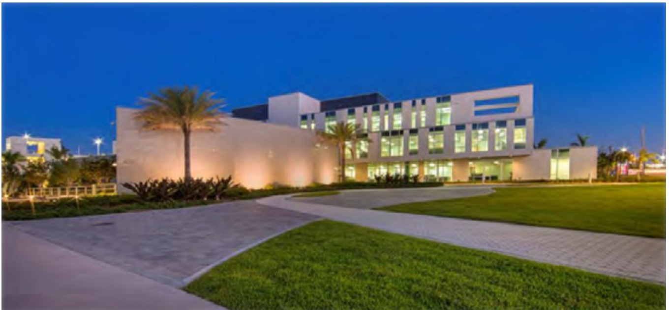
Image: City of Miami Gardens Municipal Complex
